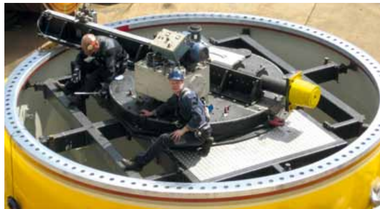
03 Flexible service on site.
