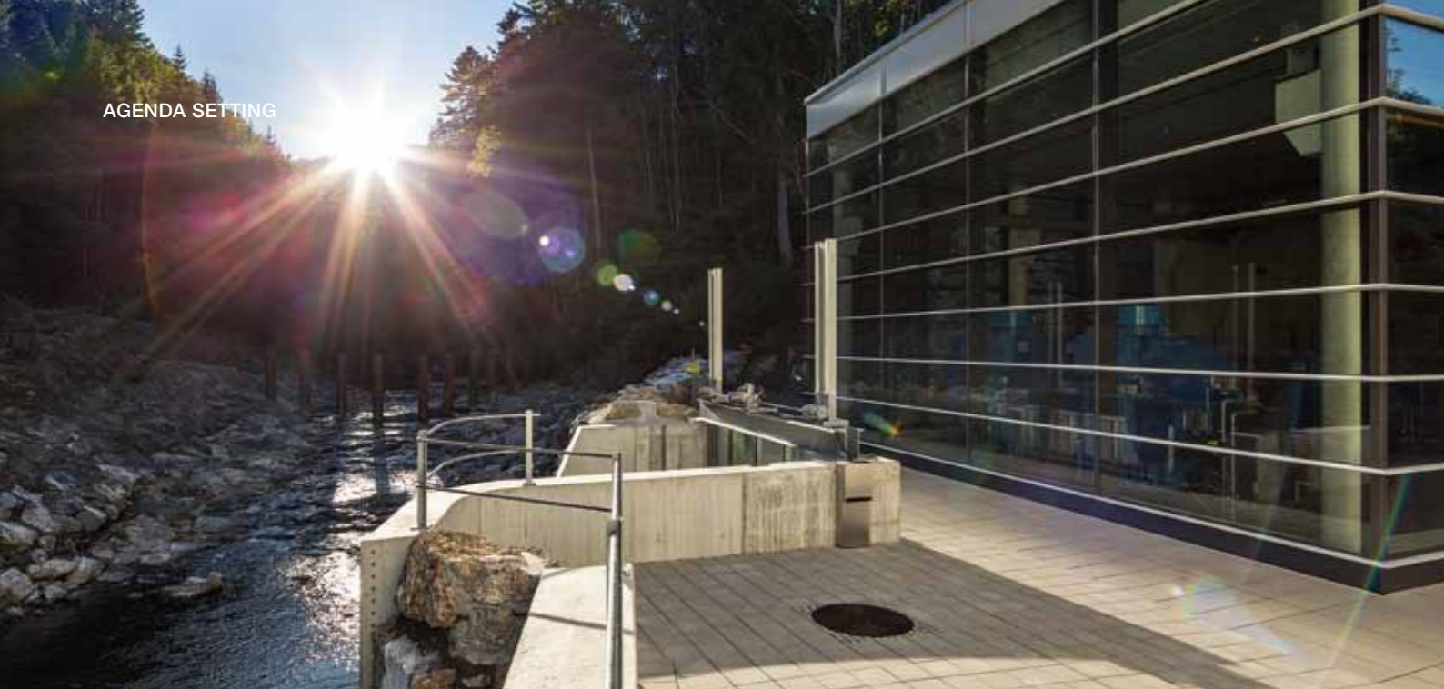
This small hydro plant in Blaichach, Germany, features an eco-friendly instream flow drain.
