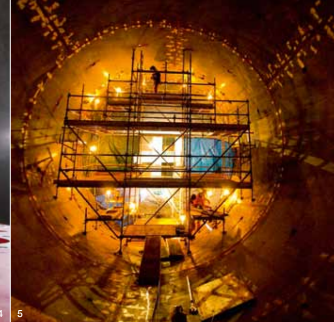
4 Inspecting a new equipment arrival: Marc Gagnon standing inside one of the head covers. 5 Workers inside the scroll case, which is almost as large as an underground train tunnel.
