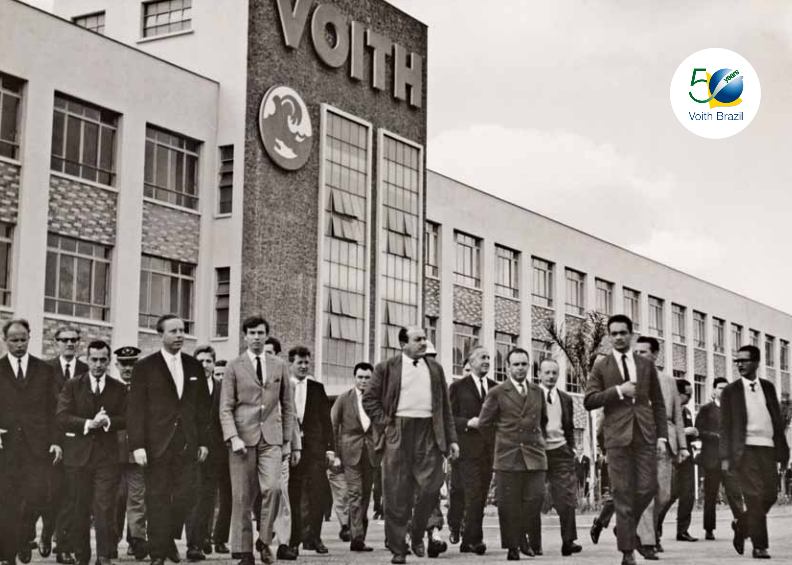
The beginning: opening of the Voith facility at São Paulo in 1966.
