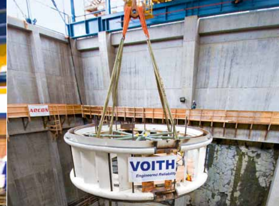
The stay ring is lowered to the turbine floor.
