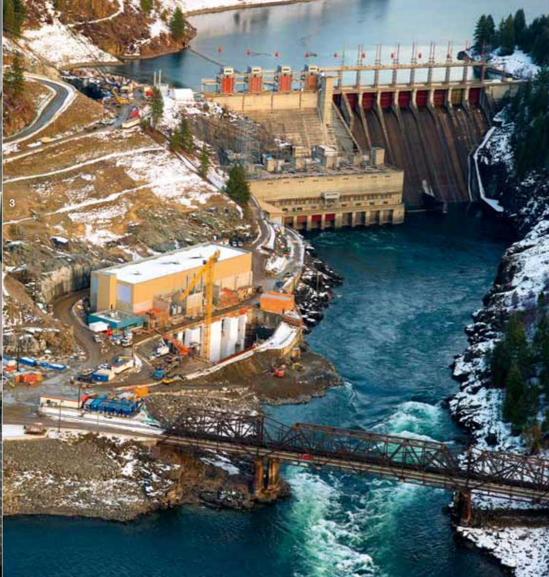
1 Detail of a turbine runner being installed at Waneta. 2 Working on the stator of Unit 2 of the Waneta plant. 3 An aerial view of the Waneta Expansion Project on the Pend d'Oreille River.
