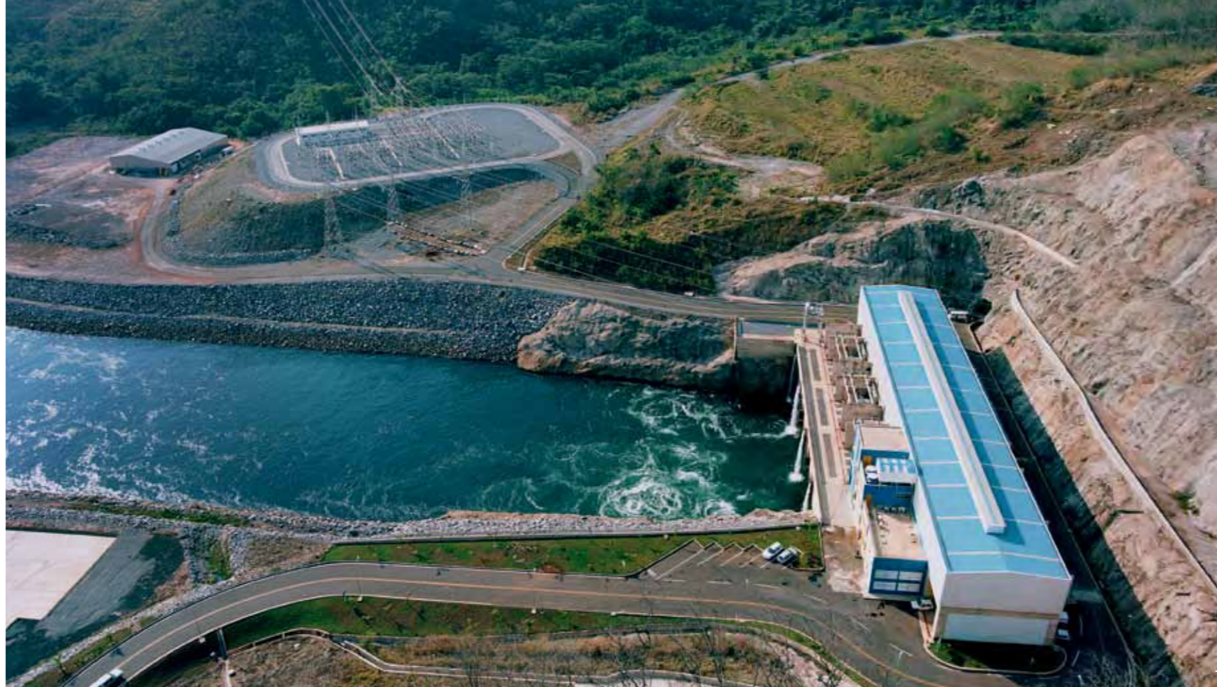
1 Capim Branco power station, Brazil. 2 Cross-functional teams ensure an optimal result. 3 Smart plant construction.
