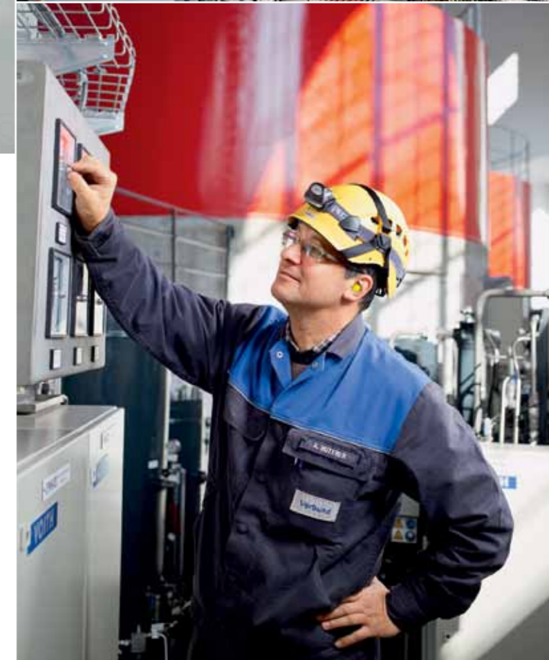
Control room and equipment
