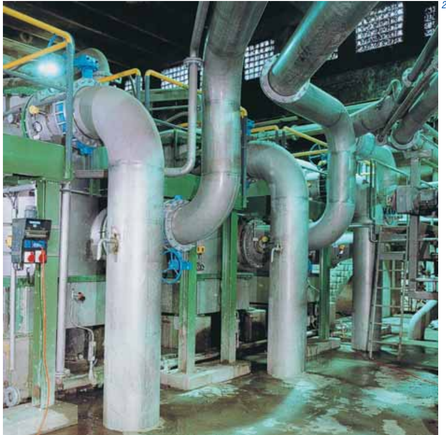
Fig. 2: Slotted fine screening system.
