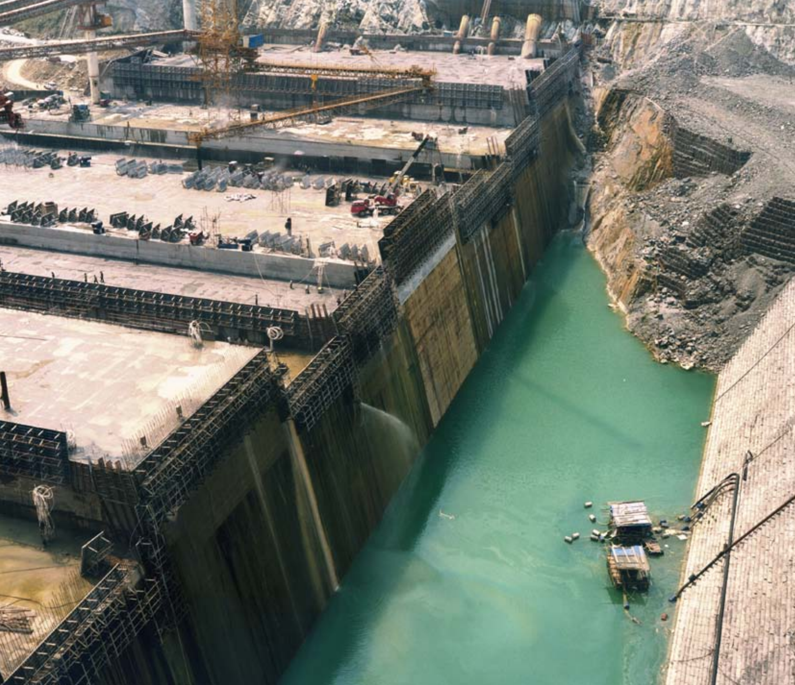
Construction of the Long Tan power plant on the Hongshui river.
