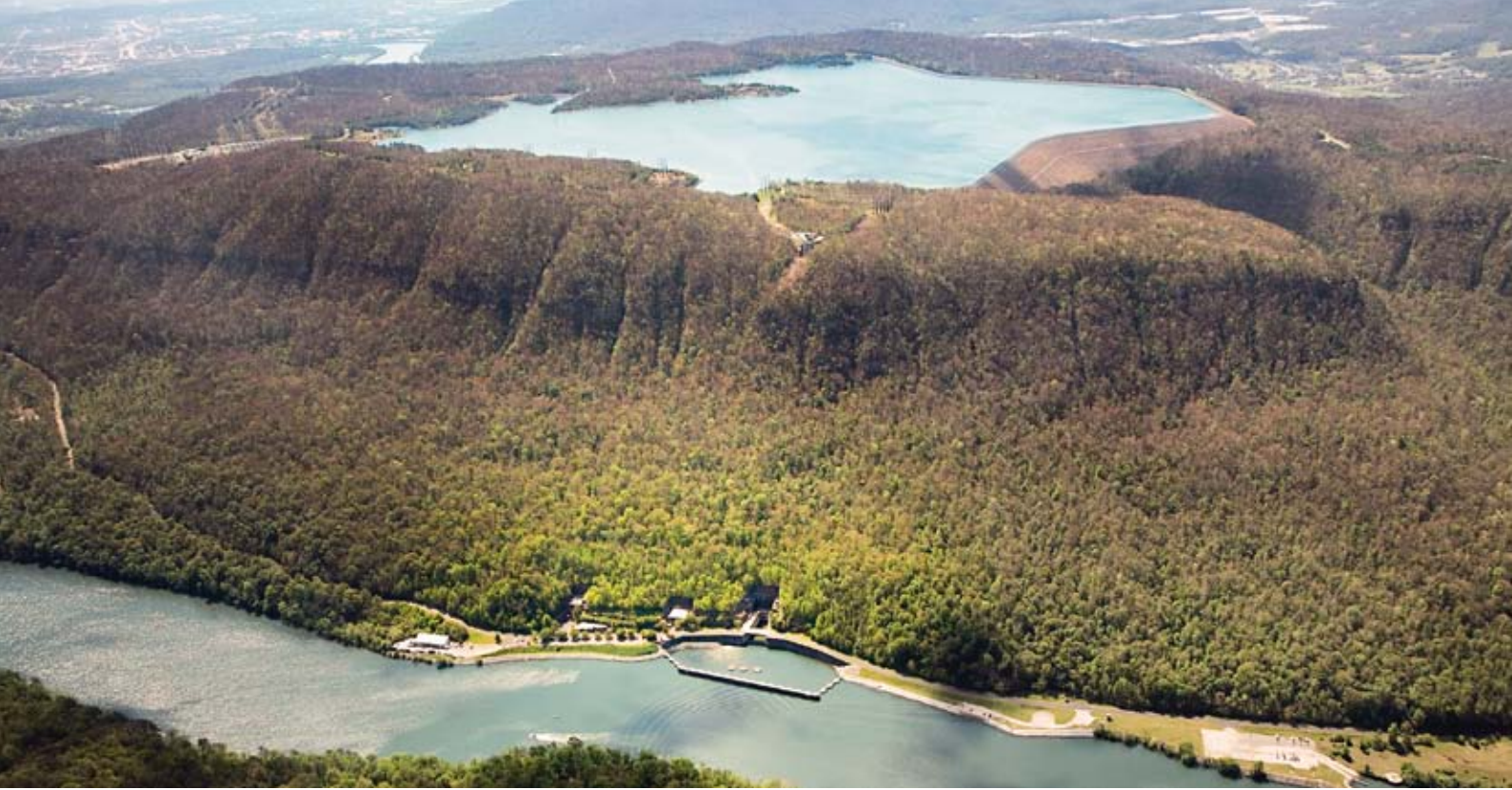
View of the Raccoon Mountain pumped storage plant on the Tennessee River.
