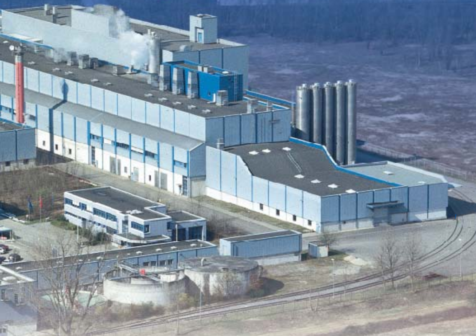
Fig. 1: The Kehl plant of August Koehler AG, showing the new PM 6 building in the left foreground.
