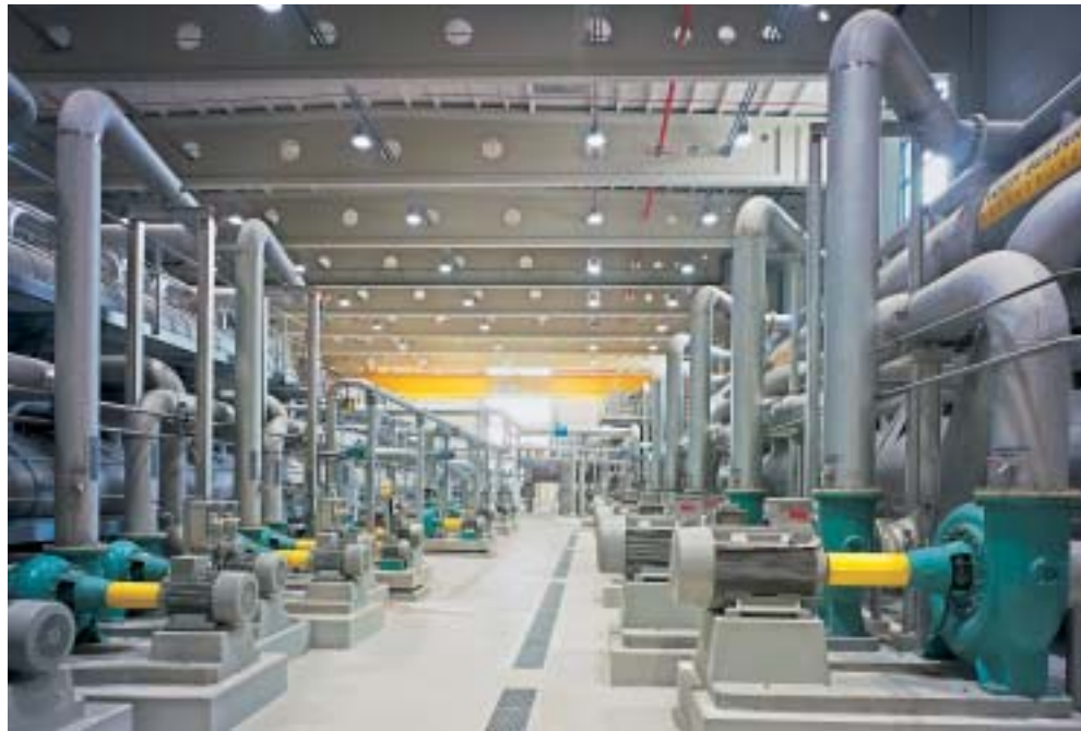
Fig. 4: Flotation I and II: primary cells on the right, secondary cells on the left with stickies flotation. Service accessibility of the entire line is exceptionally good.
