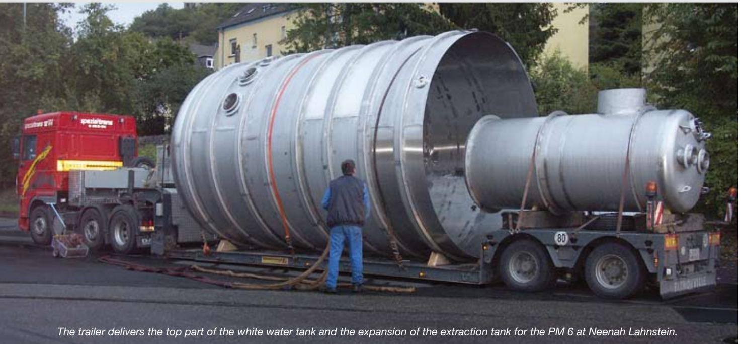
*The trailer delivers the top part of the white water tank and the expansion of the extraction tank for the PM 6 at Neenah Lahnstein.*
