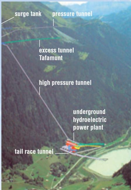
Kopswerk II will share the Kops storage reservoir with the existing plant. The upper reservoir is approximately 1,800 meters above sea level. The new headrace tunnel to be built is an approximately 5,500 meter-long pressure tunnel (4.60 - 5.30 meters in diameter) and will lead to the Tafamunt surge tank. From there it is led through a 1,380 m long pressure tunnel (3.80 meters in diameter) to the distributing conduit and pumped-storage cavern.
