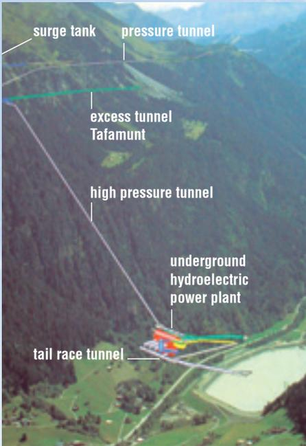
Kopswerk II will share the Kops storage reservoir with the existing plant. The upper reservoir is approximately 1,800 meters above sea level. The new headrace tunnel to be built is an approximately 5,500 meter-long pressure tunnel (4.60 - 5.30 meters in diameter) and will lead to the Tafamunt surge tank. From there it is led through a 1,380 m long pressure tunnel (3.80 meters in diameter) to the distributing conduit and pumped-storage cavern.
