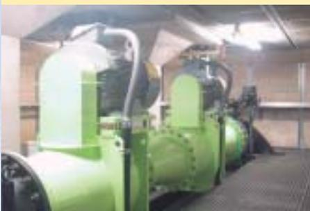
*Micro tubular turbine installed on Egasaki Drinking Water Treatment Plant (Serial arrangement of 2 units).*
