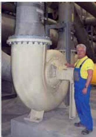
Fig. 2: High-efficiency LEF pump.
