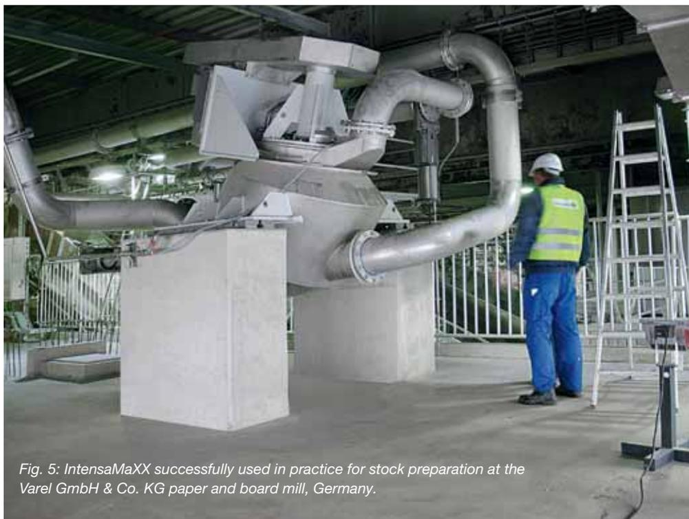
Fig. 5: IntensaMaXX successfully used in practice for stock preparation at the Varel GmbH & Co. KG paper and board mill, Germany.
