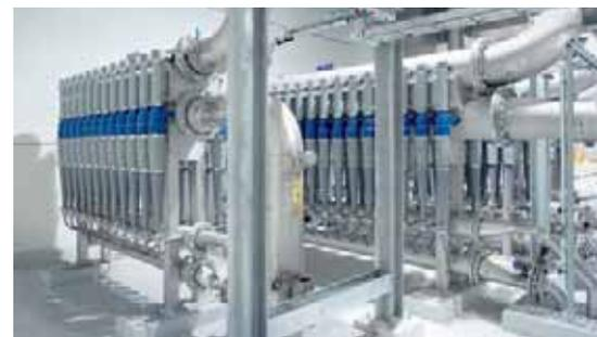
02 The new HiClean facility in the approach flow system of Perlen Papier's PM 7 in Switzerland results in lower energy costs and enhanced flexibility with respect to grade changes.
