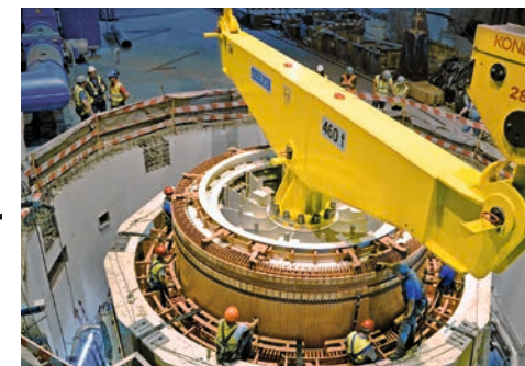
One of the asynchronous motor-generator units being installed at Frades II.
