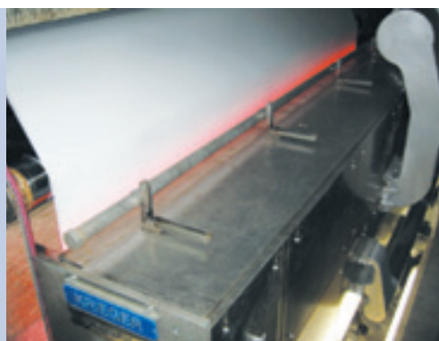
InfraAir dryer after installation.
