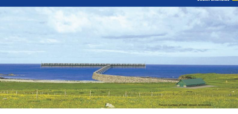
It will not only be deployed in the Siadar scheme but in future wave energy projects worldwide. It applies Voith Hydro Wavegen's oscillating water column technology and was developed with support from the Scottish Government's Wave and Tidal Energy Support (WATES) scheme.
