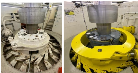
The original 1950s turbine (left) has been replaced by a new Voith turbine (right).
