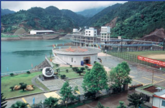
Pumped storage plants have been developed as “energy storage systems” capable of quickly responding to fluctuations in power demand. In times of reduced energy demand, excess electric capacity in the grid is used to pump water, previously used to generate power, back into an upper reservoir. This water can then be used to generate electricity when needed.
