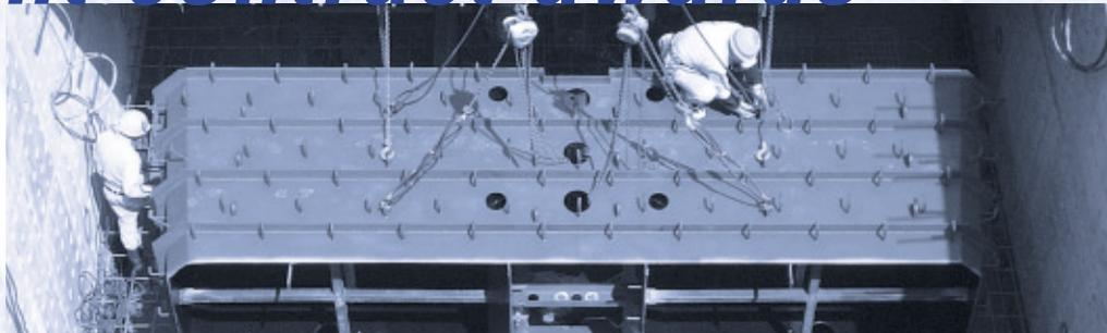
*Final assembly of the draft tube liner before embedment at Tomada hydro power station.*
