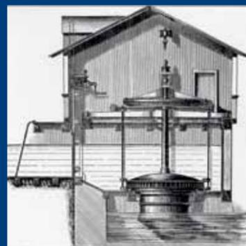
The first water turbine from Voith: a 100-horsepower Henschel-Jonval turbine
