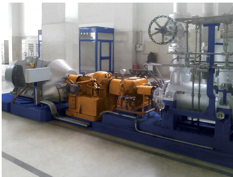
Figure 1: The Voith variable speed fluid coupling (type 510 SVL) has been operating reliably since 1956 without unplanned downtime.
