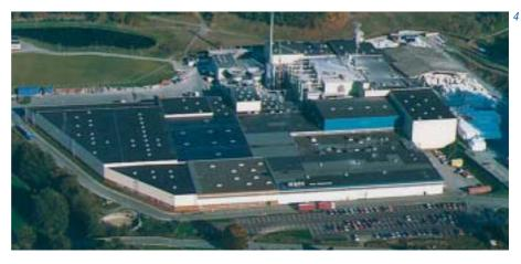
for a speed of 2200 m/min. At the Giershagen mill *(Fig. 4)* there are two tissue machines and a fourdrinier machine on which towels and crêped papers are manufactured. While the fourdrinier machine has a maximum speed of 920 m/min, speeds of 1600 to 1900 m/min are normal on the tissue machines.
